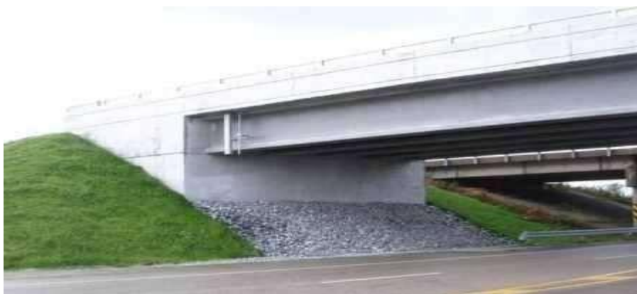
Fig 1. 4: Integral Bridge with Bank Pad Abutments
