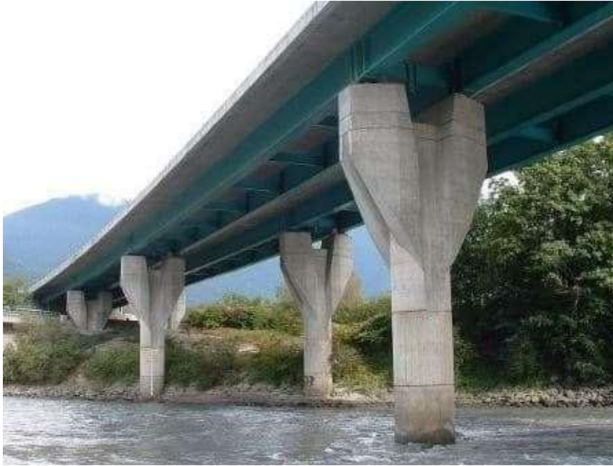
Fig 1. 6: Intermediate Supports of Integral Bridge
