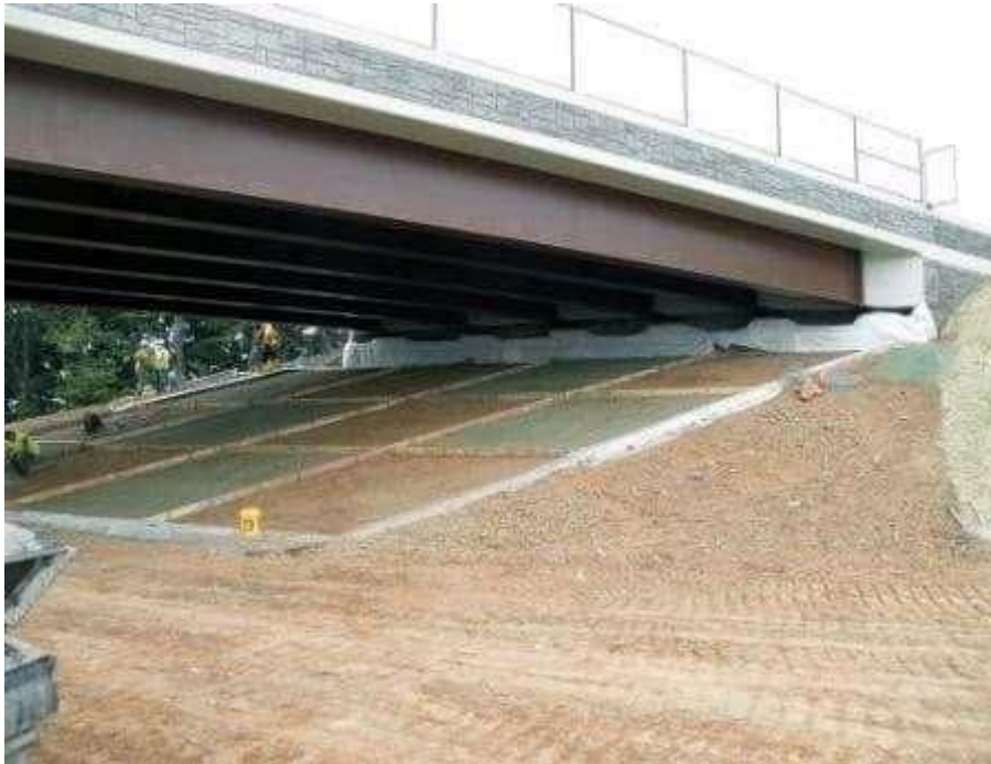
Fig 1. 5: Integral Bridge with End Screen Abutments
