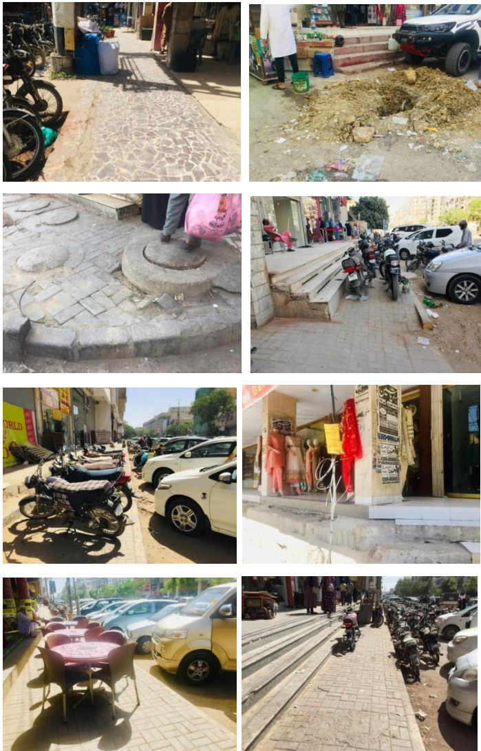
Fig 17-25: Sidewalk issues of Study Area 3. Source (Author)
