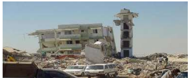
Fig. 1: collapse in bhuj (2001)
