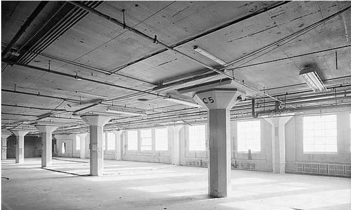
Fig 1 Flat Slab
